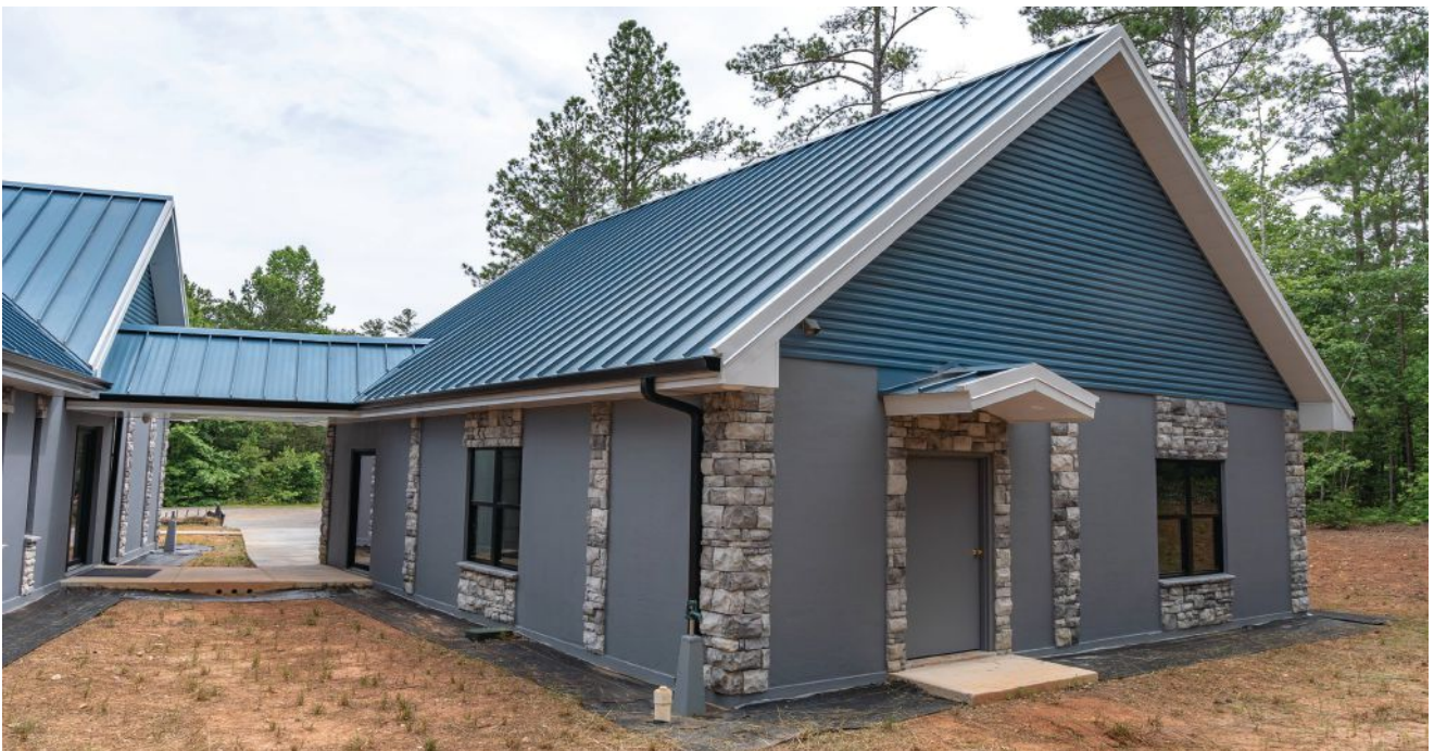
Traditional concrete homes typically offered limited architectural design options. Nonquit Homes' premier installation, combining painted precast concrete panels with siding and manufactured veneer stone accents, shows how the industry has come a long way.
