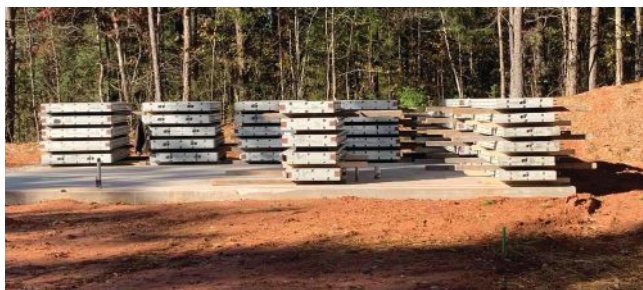
Nonquit Homes schedules wall panel fabrication, stressing and staging after main home and garage slabs can bear crew, formwork and forklift loads.
