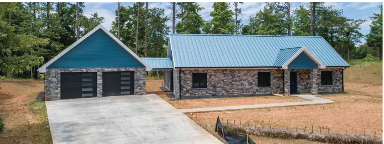
Traditional concrete homes typically offered limited architectural design options. Nonquit Homes' premier installation, combining painted precast concrete panels with siding and manufactured veneer stone accents, shows how the industry has come a long way.
