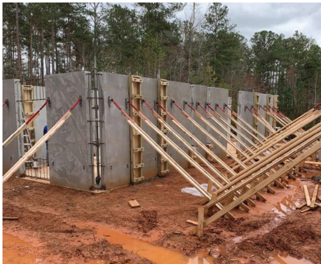
Nonquit Homes schedules wall panel fabrication, stressing and staging after main home and garage slabs can bear crew, formwork and forklift loads.
